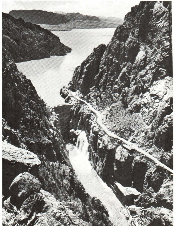
Buffalo Bill Dam, Wyoming, provides for irrigation of the Shoshone Valley.
