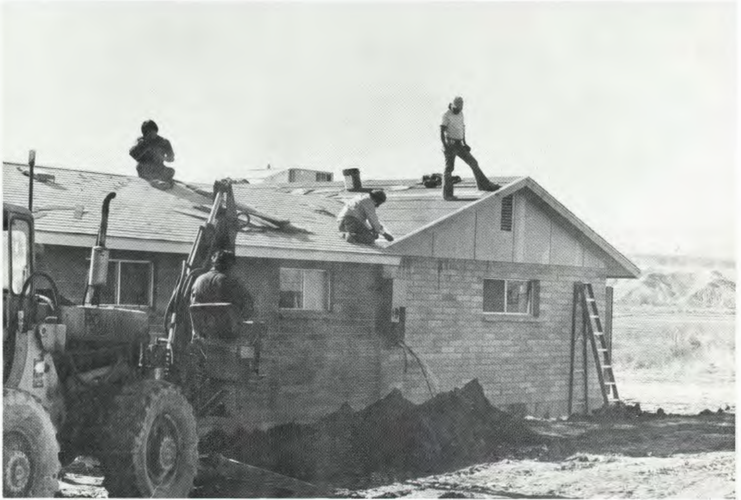
CONSTRUCTION CREW AT WORK
