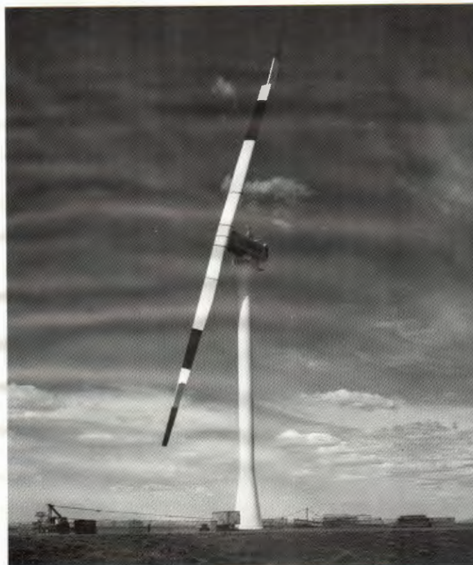
The MOD-2 wind generator at Medicine Bow, Wyoming
