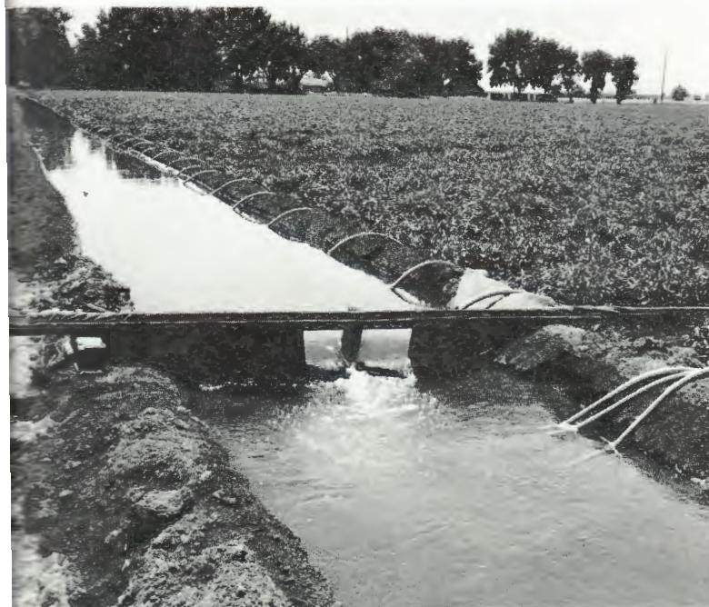
Irrigation project, Solano County, California.
