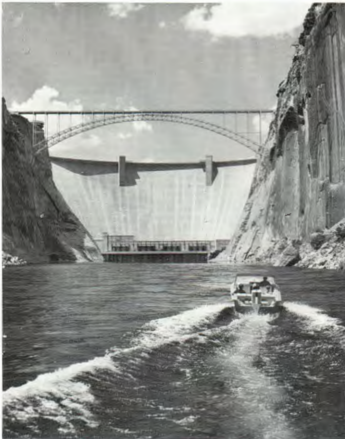
Glen Canyon Dam, Utah-Arizona.
