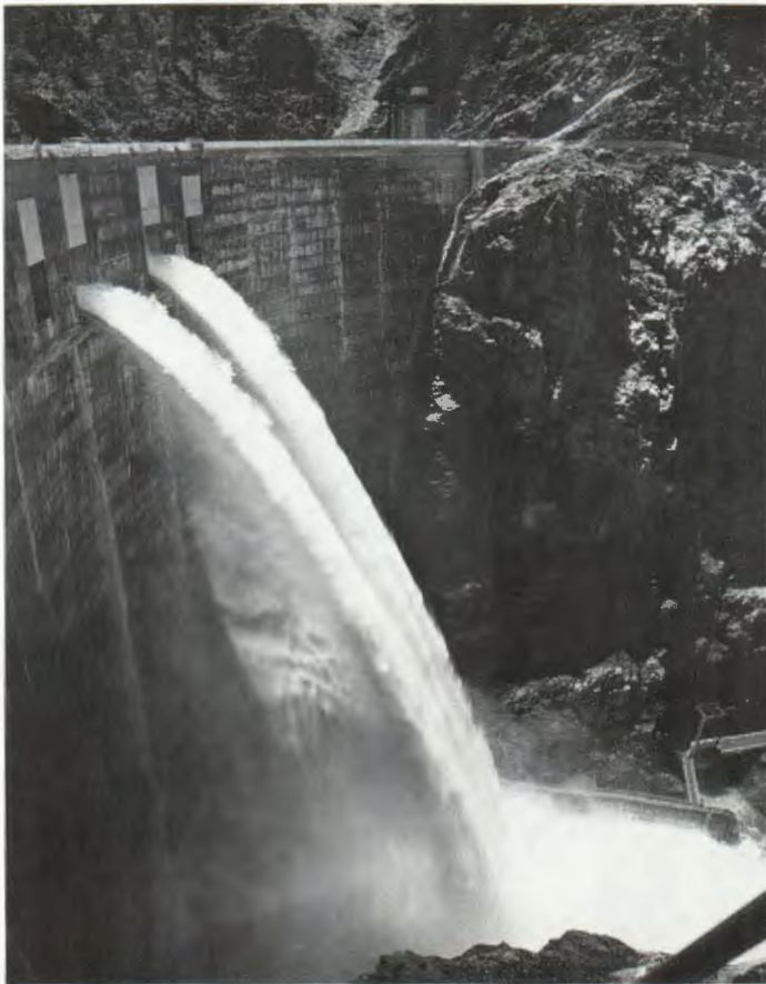
High water flows at Morrow Point Dam, Colorado River Storage Project, in 1983. Bureau of Reclamation flood control efforts help protect life and property.
