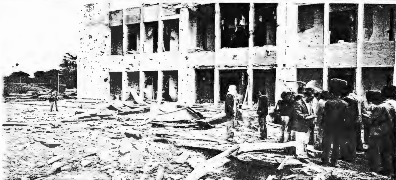
Payoff: the shattered façade of Gaddafi's headquarters in Bab al Azizia army compound on the day after the attack
