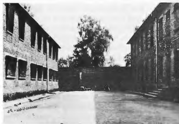
The execution wall at Auschwitz. On close examination the imprint of agonized fingers are evident in the brick. [photo credit: YIVO]
