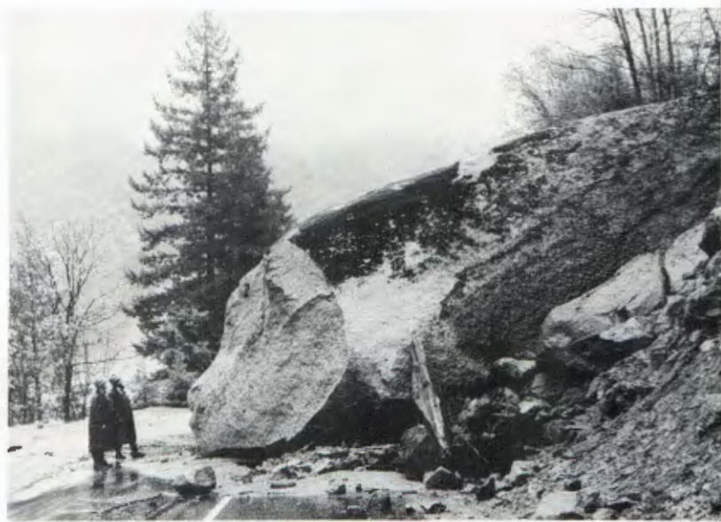
Although The Ahwahnee wasn't damaged by the great flood of December, 1937, boulders blocked roads! (Ansel Adams photograph; SS Collection.)
