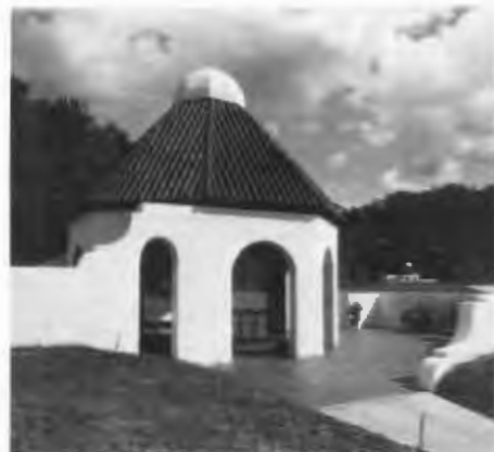
Committal shelters built by cemetery labor at Puerto Rico National Cemetery.
