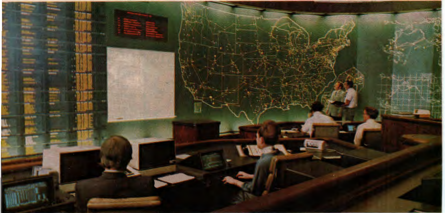
The Network Operations Center, Bedminster, New Jersey.
