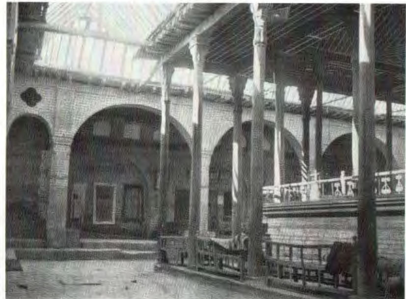
Plate 13. The new synagogue, Baghdad. The space between the sides and the centre of the synagogue is not covered. Built in 1797, on the site of a much older synagogue, by permission of Suleiman Pasha, Vali of Baghdad. Renovated 1854-55. Near the entrance of another synagogue, the Great Synagogue, was a stone set in the wall with the inscription 'a stone from the land of Israel' which was touched with the fingers on entering and leaving, and which had been brought from Palestine in 1868.
