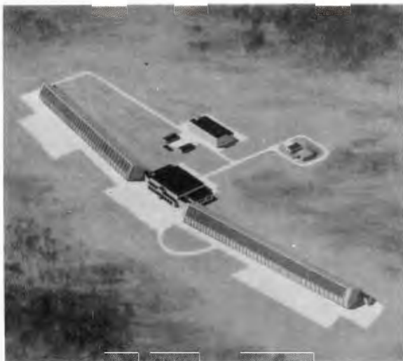
HEN HOUSE ballistic missile early warning radar
