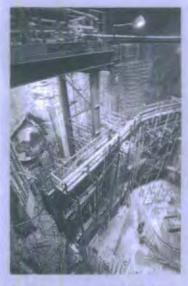
▲ Dillingham built PG&E's 140 MW Kerckhoff Hydroelectric Power Project, including one of the largest silo-type underground powerhouses in the world and a machine-bored 24 foot-diameter by 22,000-foot-long tunnel, all in granite — monumental tasks that would test the mettle of any contractor. Dillingham finished six months ahead of schedule.
