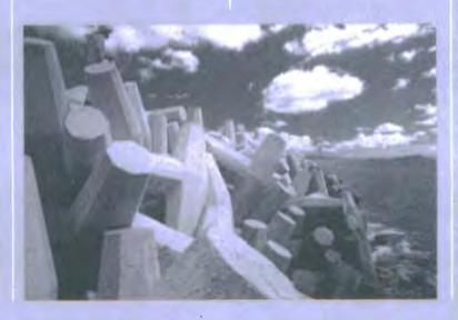
Dillingham construction of the Honolulu Reef Runway created a new land area bigger than Waikiki by dredging up 19,000,000 cubic yards of coral, protecting it with 800,000 tons of revetment rock and 18,100 concrete dolosses
