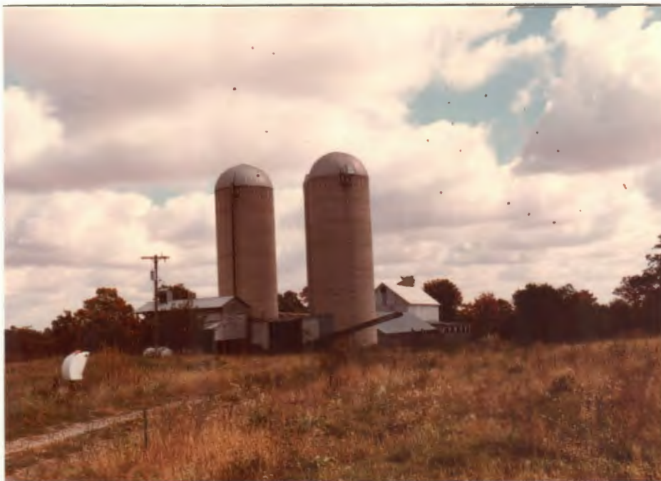
View looking northeasterly toward concrete silos.
