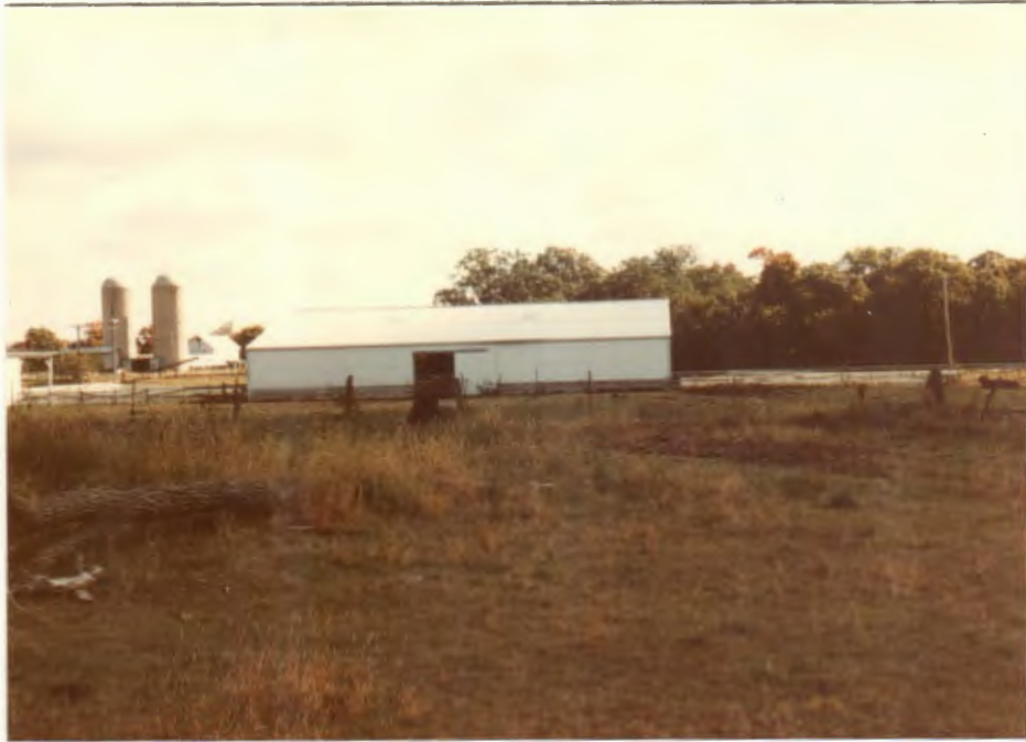
View of cattle shed.
